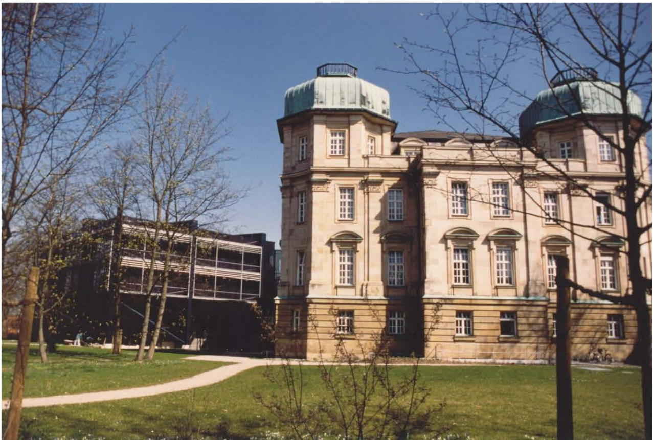
Rear facade of the Federal Supreme Finance Court
